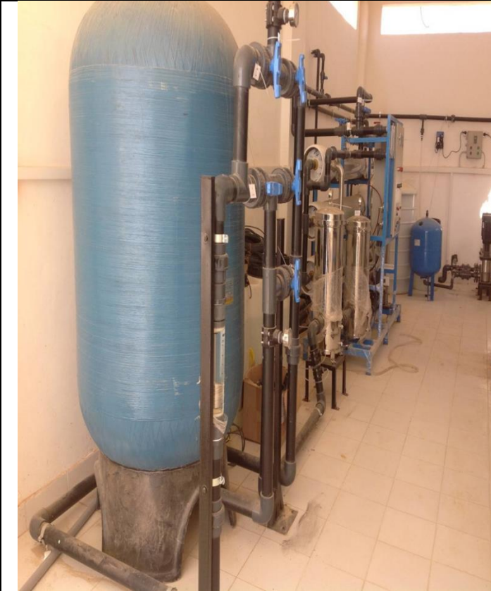
100 m 3 Desalination Unit, Wadi El-Natroom (Faculty of Agriculture, Alexandria University)
