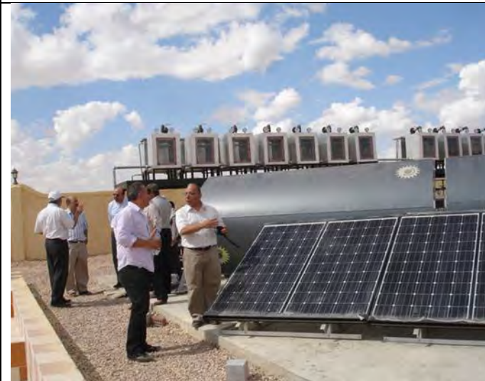
Innovative Renewable Energy (RE) Driven - Multi Stage Flash (MSF) System with Salts Precipitator and Nano Filtration (NF) Feed Water pre Treatment (RE-NF-MSF). (Faculty of Agriculture, Alexandria University)
