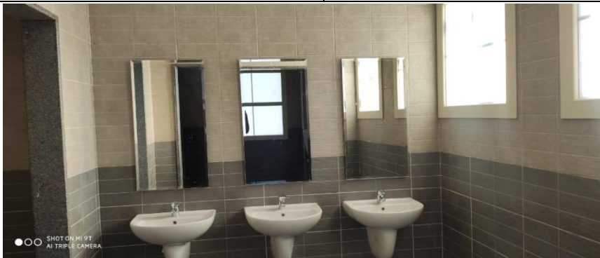
Supplying water taps with water conservation units (Alexandria University, Egypt)
