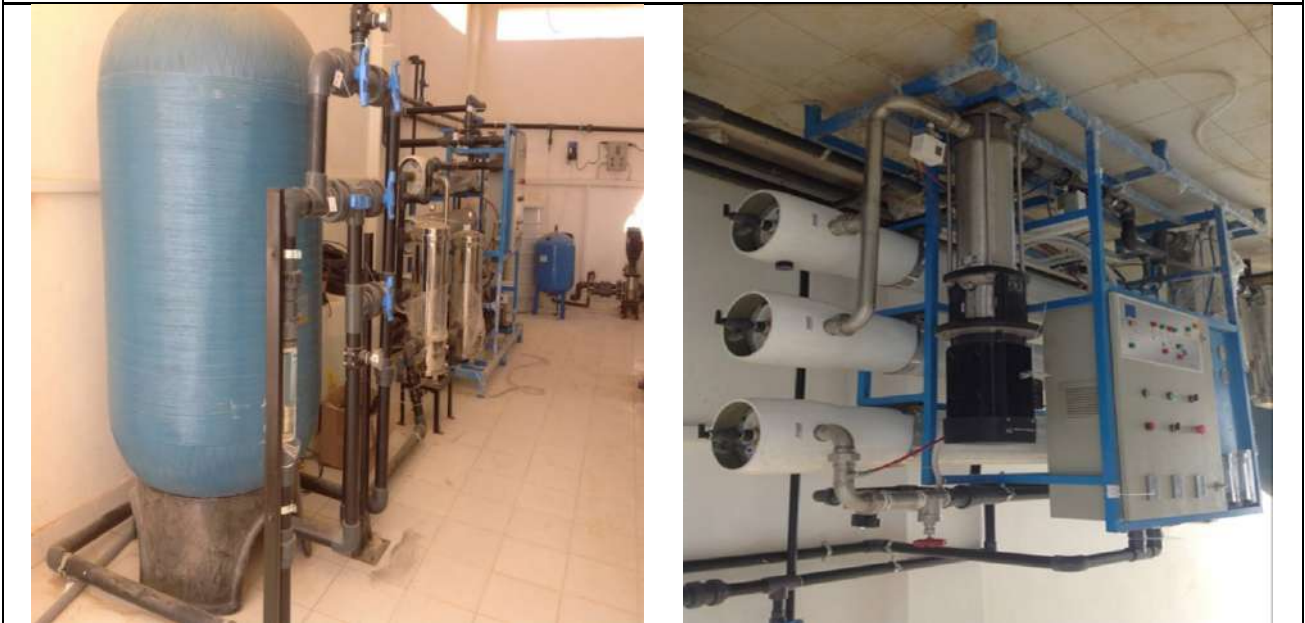
A 100 m 3 desalination unit in Wadi Natroun (Faculty of Agriculture, Alexandria University)
