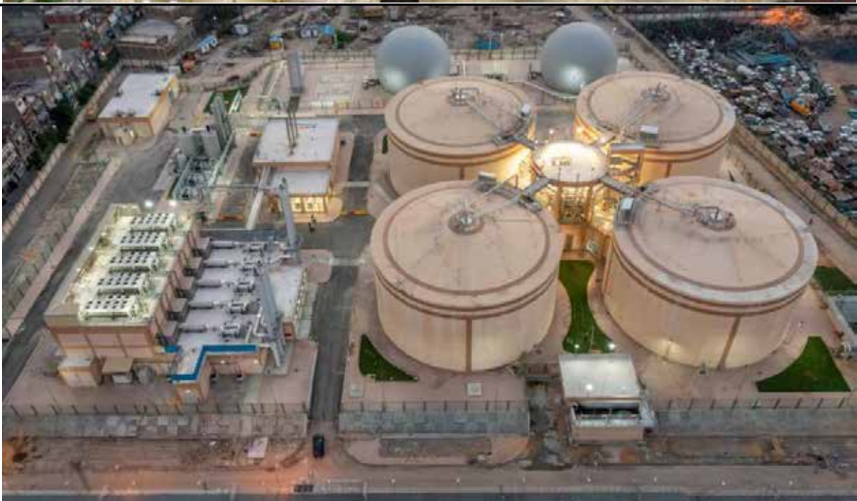
Second treatment of Alexandria University Sewage by Alexandria Sanitation Company
