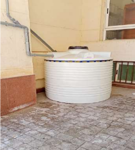
Air conditioning water collection and reuse unit - Faculty of Engineering
