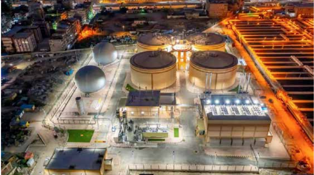
Second treatment of Alexandria University Sewage by Alexandria Sanitation Company
