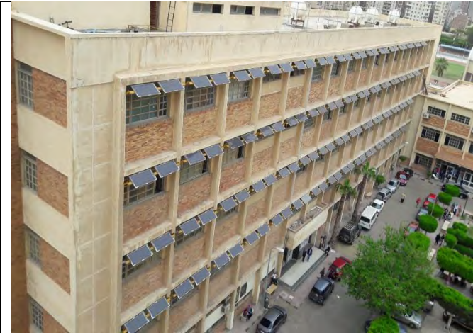
BIPV Façade Brise-Soleil System Solar Energy Project at the Faculty of Science (Alexandria University)
