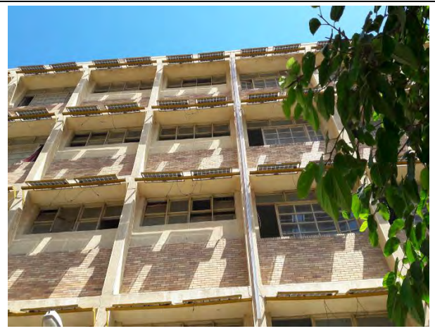
BIPV Façade Brise-Soleil System Solar Energy Project at the Faculty of Science (Alexandria University)
