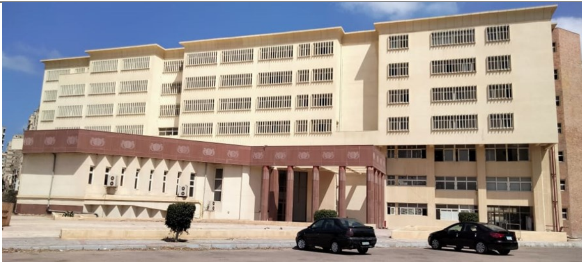
Green building implementation through the use of sun breakers in the SSP building at the Faculty of Engineering
