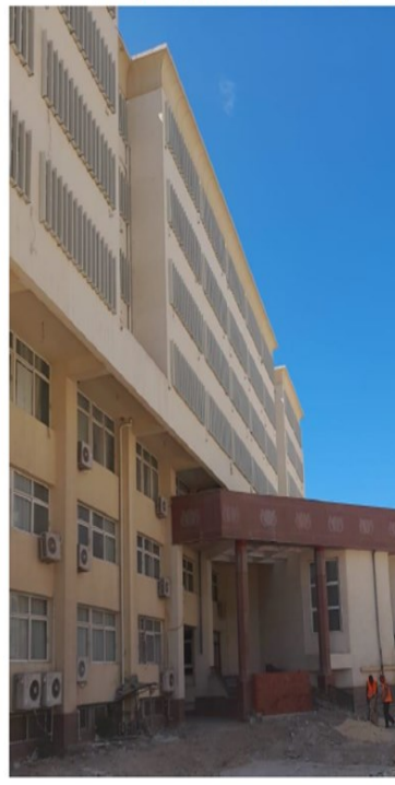
Photos of Faculty of Engineering SSP Building
