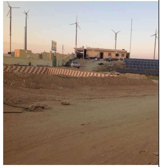
100 KW Hybrid Wind/PV System (50 KW PV and 50 KW Wind)
