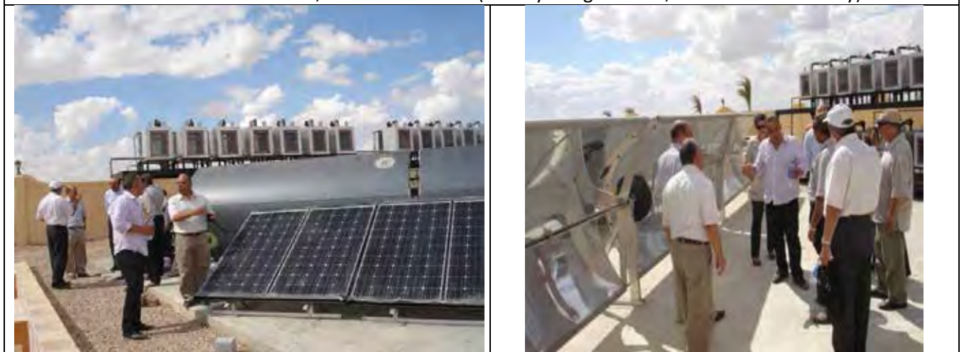
Innovative Renewable Energy (RE) Driven - Multi Stage Flash (MSF) System with Salts Precipitator and Nano Filtration (NF) Feed Water pre Treatment (RE-NF-MSF). (Faculty of Agriculture, Alexandria University)
