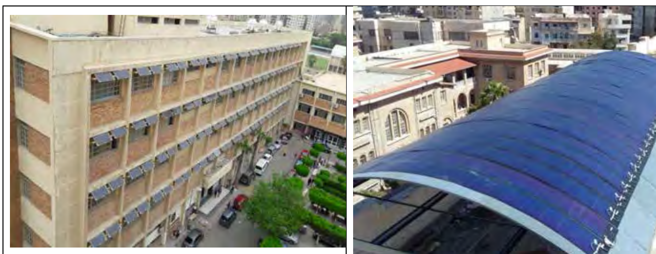
BIPV Façade Brise-Soleil System Solar Energy Project at the Faculty of Science (Alexandria University)
