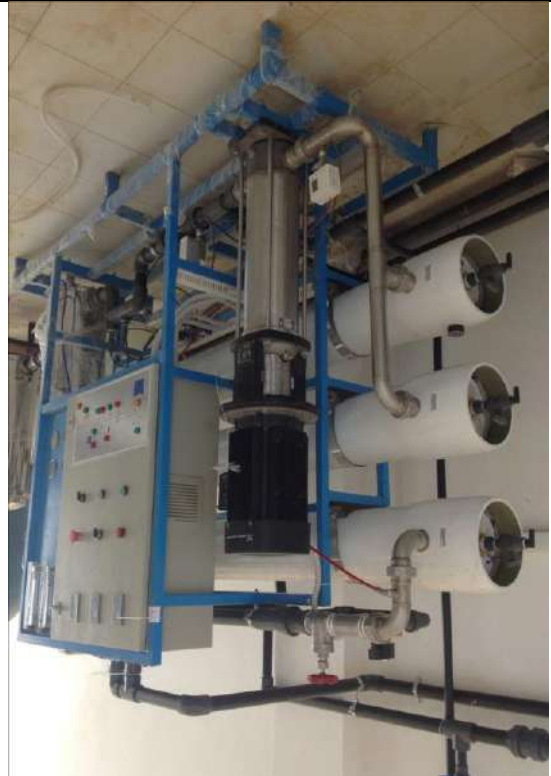
100 m3 Desalination Unit, Wadi El-Natroom (Faculty of Agriculture, Alexandria University)
