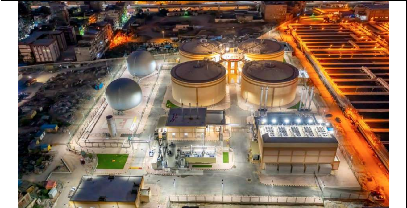
Second treatment of Alexandria University Sewage by Alexandria Sanitation Company
