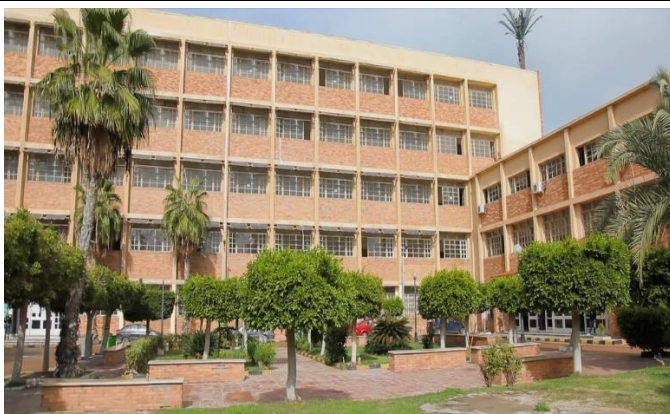
Pedestrian path and street lamp for pedestrian in night (Alexandria University, Egypt)
