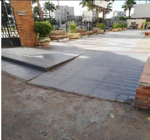
Replacing steps with ramps for disabled people (Faculty of Pharmacy - Alexandria University)
