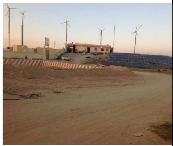
100 KW Hybrid Wind/PV System (50 KW PV and 50 KW Wind)
