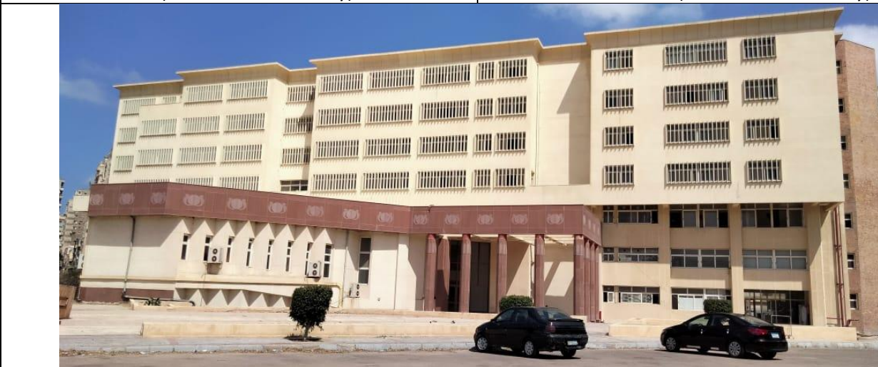
Green building implementation through the use of sun breakers in the SSP building at the Faculty of Engineering
