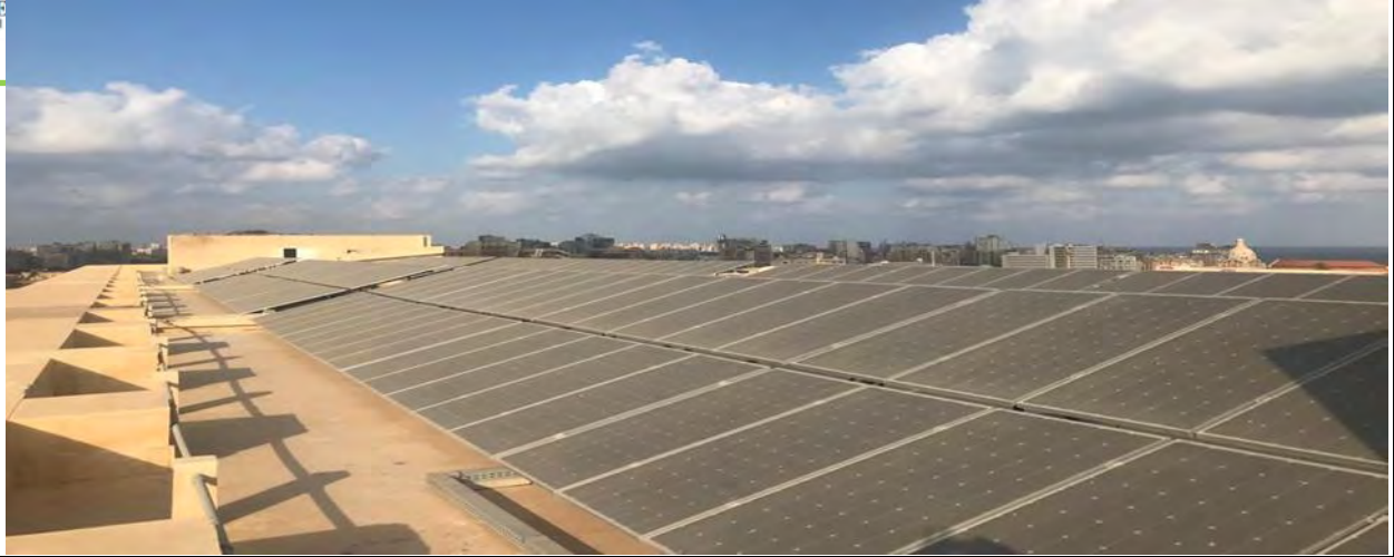
Solar photovoltaic with a capacity of 220 kilowatts on the 2000 m 2 roof top of the building of the Mechanical Engineering Department at the Faculty of Engineering (Alexandria University, Egypt)
