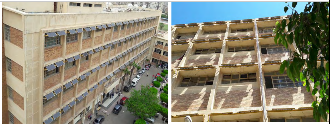
BIPV Façade Brise-Soleil System Solar Energy Center at the Faculty of Science (Alexandria University)
