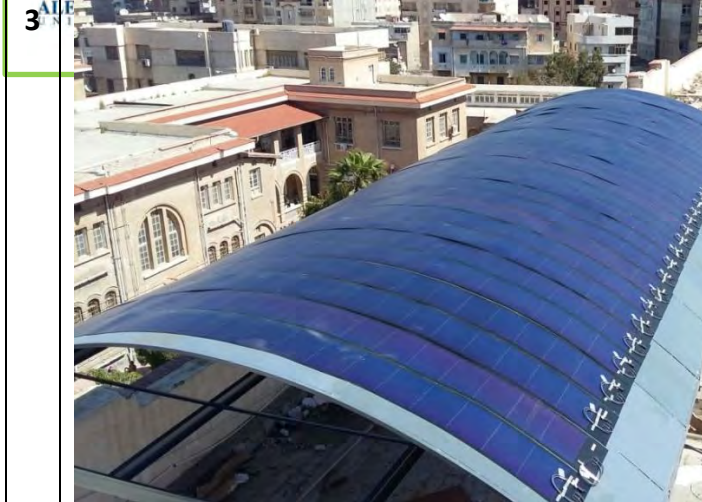
BIPV Roof Pergola, Faculty of Science in Moharram Bek (Alexandria University)
