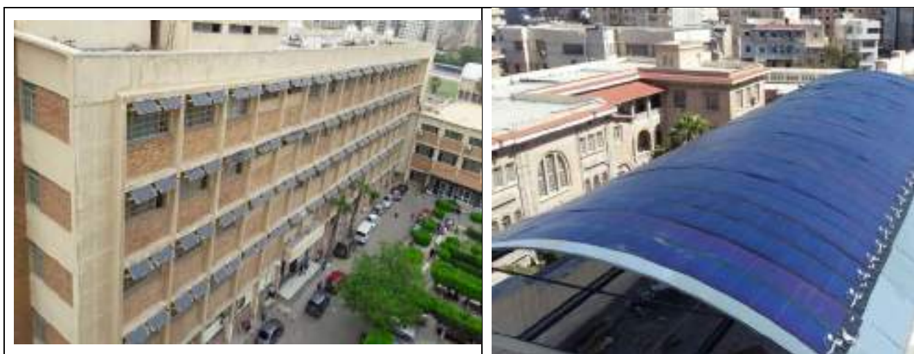
BIPV Façade Brise-Soleil System Solar Energy Project at the Faculty of Science (Alexandria University)
