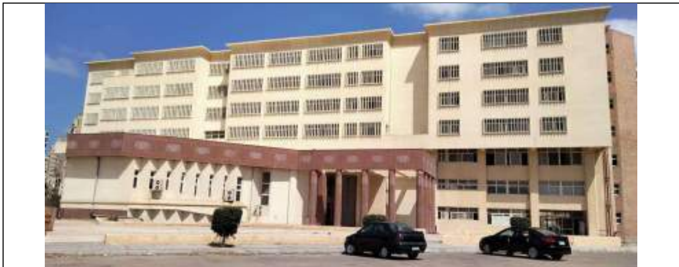
Green building implementation through the use of sun breakers in the SSP building at the Faculty of Engineering
