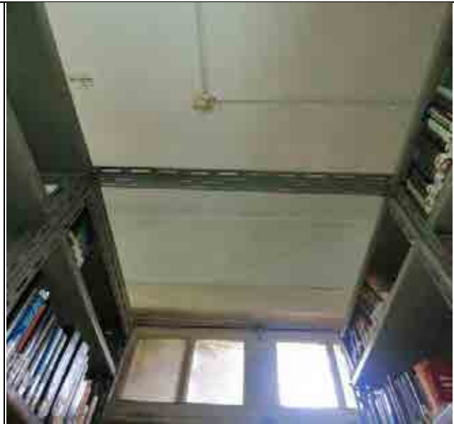
5. Fire Alarm (smoke detector)
