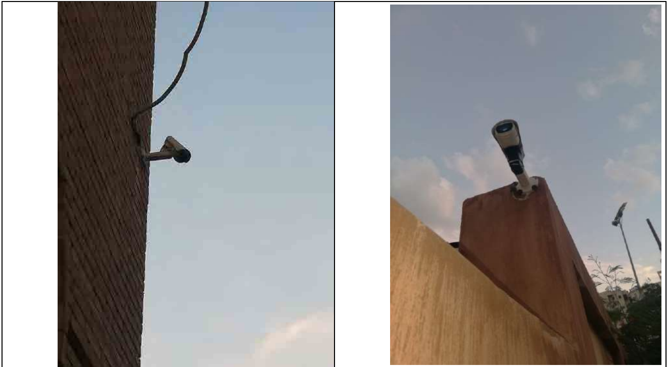
7. Video surveillance system at Alexandria University
